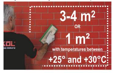
To facilitate application (especially in hot climates), you can lightly moisten the surface of the tiles with the supplied sponge squeezed before applying the product, avoiding stagnation on the surface of the tiles or in the joints that are still empty. This allows the product to be applied better, slowing the
